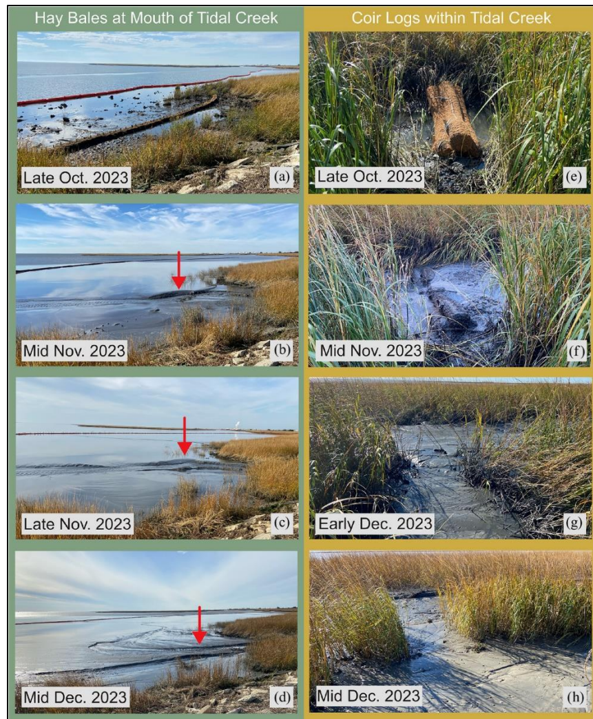
Figure 4. Roving camera images of (a–d) hay bale containment at the mouth of the tidal creek; and (e–h) coir logs within the tidal creek. Arrows denote scour.
