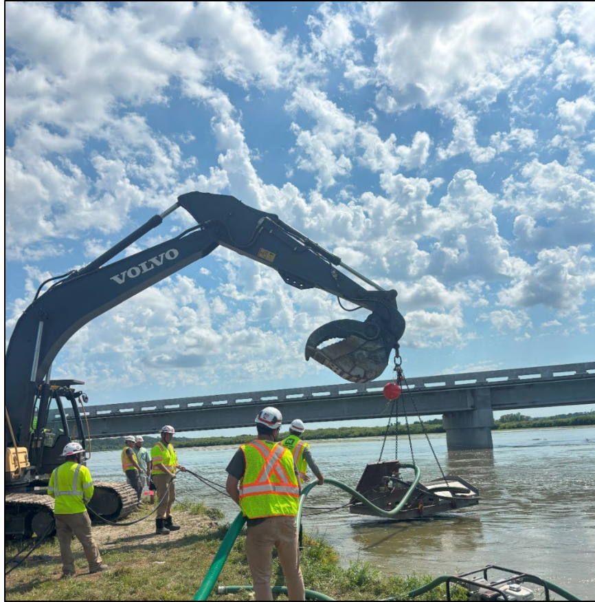
Figure 1. The 4-foot bedload sediment collector being deployed into the Niobrara River.
