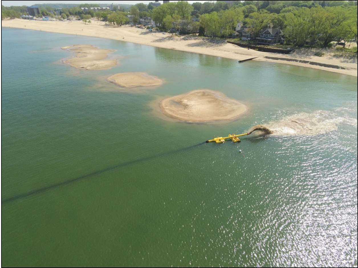
Figure 12: Dredging placement near St. Joseph harbor, photo taken by UAS.
