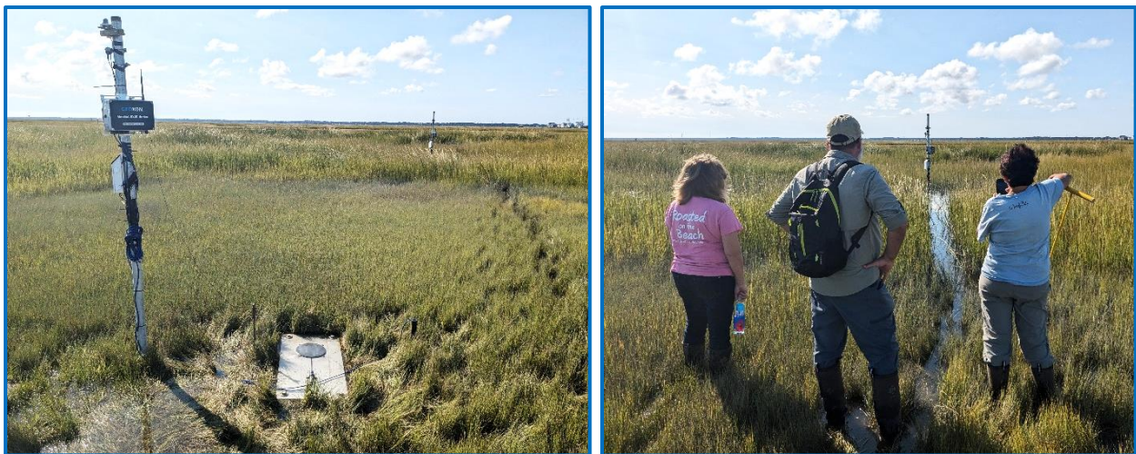
Figure 2. (Left) Final installation of the geotechnical sensors co-located with the ecological sensors at the high-marsh site. The low-marsh site can be seen in the background, right-hand side. (Right) Monica Chasten (USACE NAP), Dr. Anthony Priestas (CHL), and Dr. Lenore Tedesco (The Wetland Institute) discussing construction plans for the upcoming BUDM placement. Photos collected by Dr. Brian Harris.
