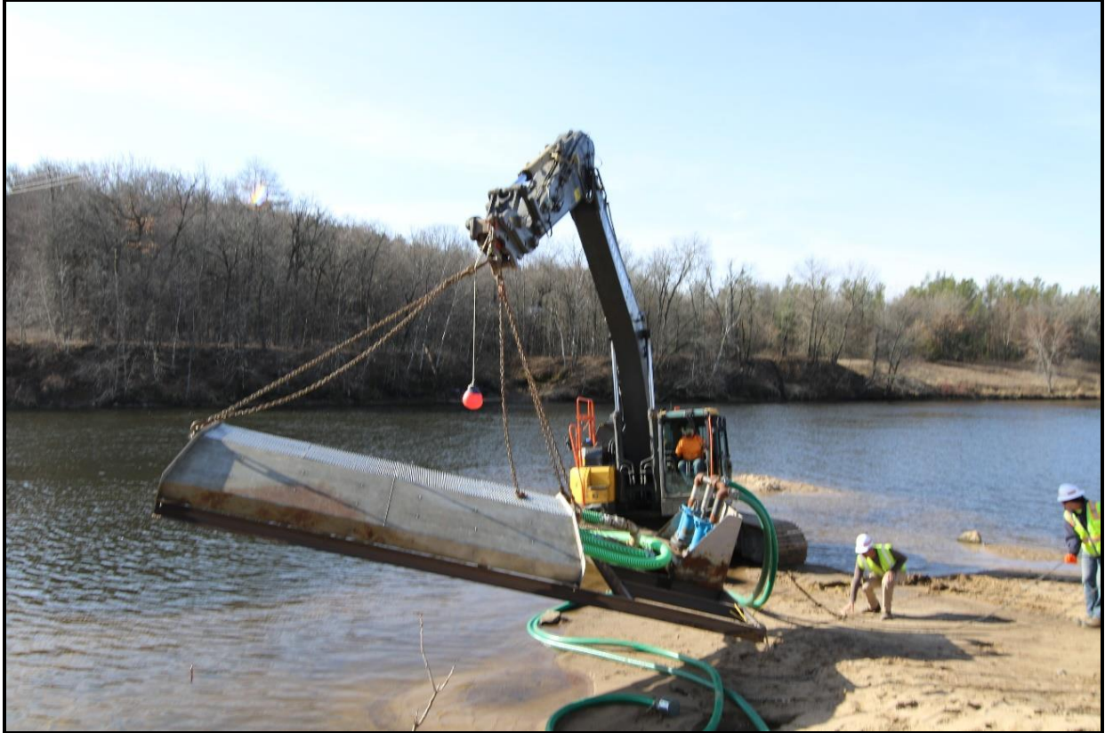
Figure 1. Bedload sediment collector being installed in the Eau Claire River, Wisconsin, 12 March 2024.
