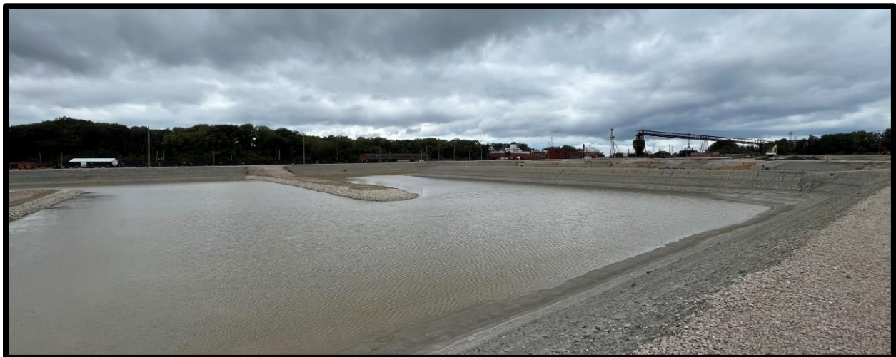
Figure 5. Conneaut Creek Dredge Reclamation Facility.
