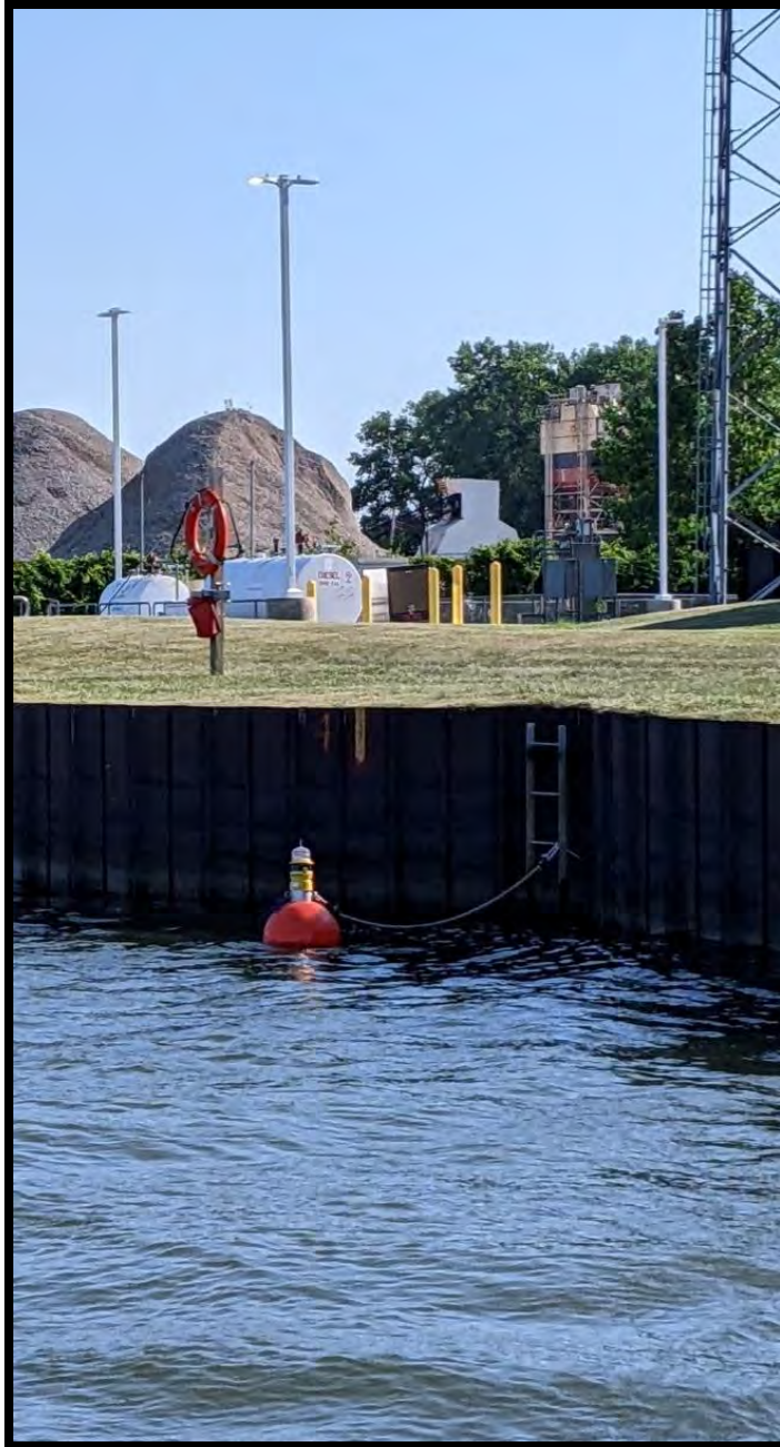
Figure 3. Placement of the eighth buoy and turbidity sensor outside the Coast Guard station at the mouth of Fairport Harbor, OH.
