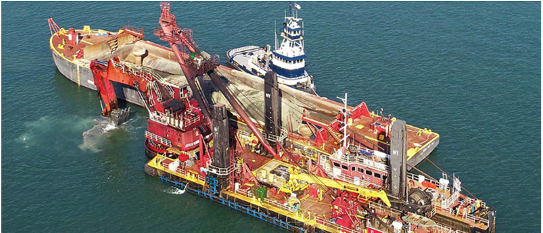
Photo courtesy of Great Lakes Dredge & Dock Company
