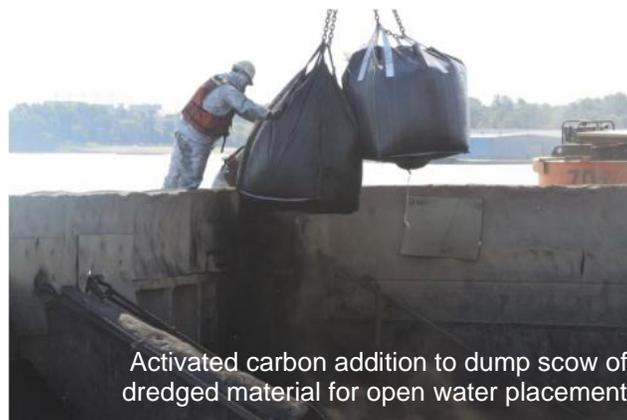
Activated carbon addition to dump scow of dredged material for open water placement
