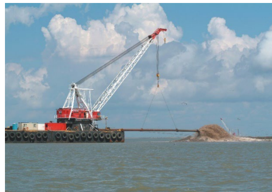
Dredge placing material at a DPA.
