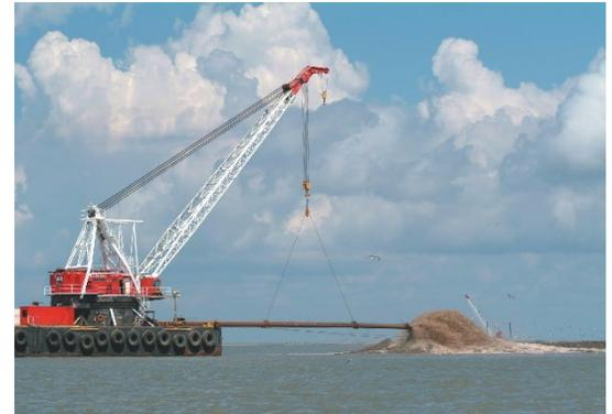
Figure 1. Dredge placing material at a DPA
