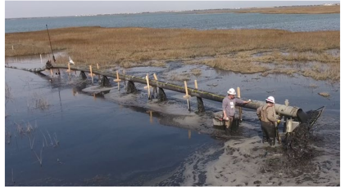
Sediment Distribution Pipe demo on Sturgeon Island March 2020
