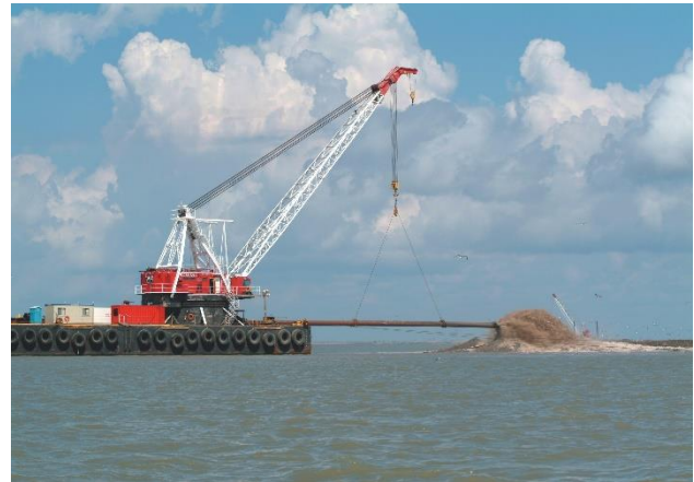
Figure 1. Dredge placing material at a DPA
