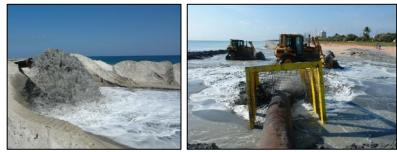
the dredging process. Methods will include collecting numerous samples of intake and pump-out material at a wide variety of locations and aboard various dredge types. This data will be used to empirically estimate the reduction in fines as a function of the amount of fines in situ as well as by dredge type used for construction.
